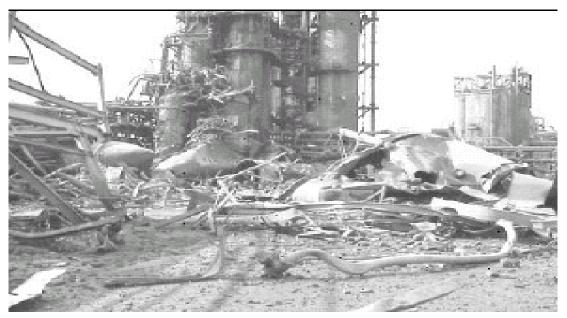
Photo of damage to bauxite plant following pressure vessel failure.
